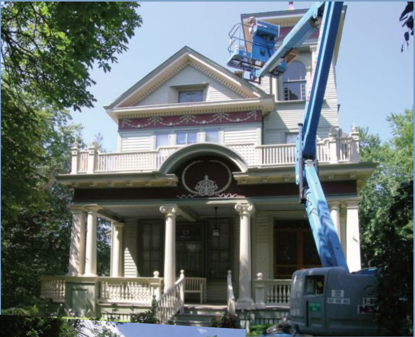
Today's neighborhood- Koenig House being restored at 1731 N. 32nd
